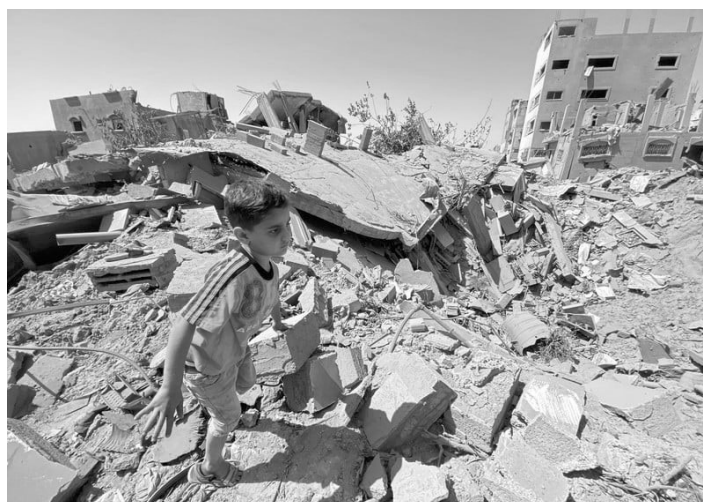
Twelve buildings are destroyed every hour in Gaza.
