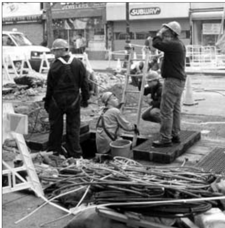
Utility workers laying new cable on Steinway Street, a normally crowded shopping hub in Astoria.
